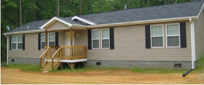
1995 – Present “modern” Base Grade C Functional Dep 0%
