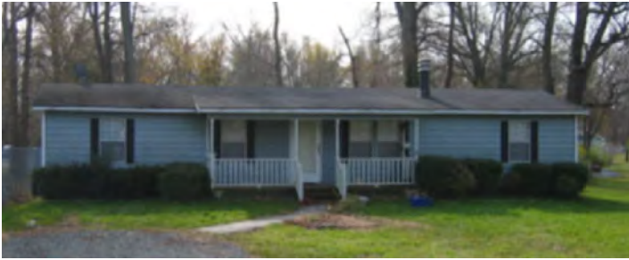
Mid-80’s – 1994 “vinyl/shingle” Base Grade C- Functional Dep 0% - 10%
